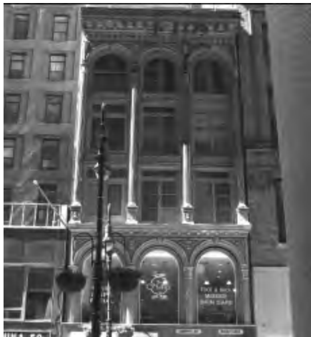
Designation as an individual landmark is being sought for 63 Nassau Street, a cast-iron-fronted building between Maiden Lane and John Street.
