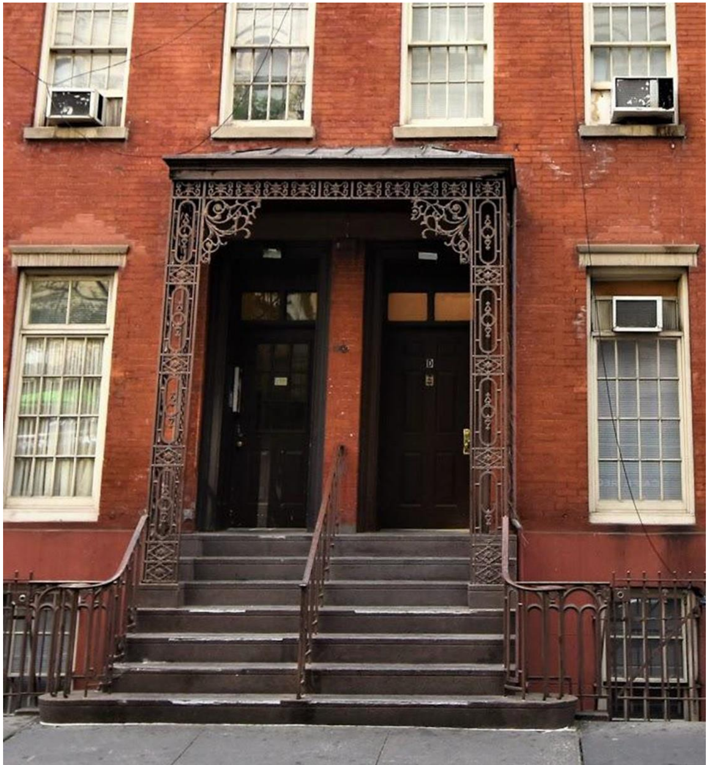
Designated landmark at 130-132 MacDougal Street, 1852, with ironwork called out in the designation report as original. Note that the corner brackets are identical to those on the ironwork at 50 West 13 th Street, and the overall character is the same.
