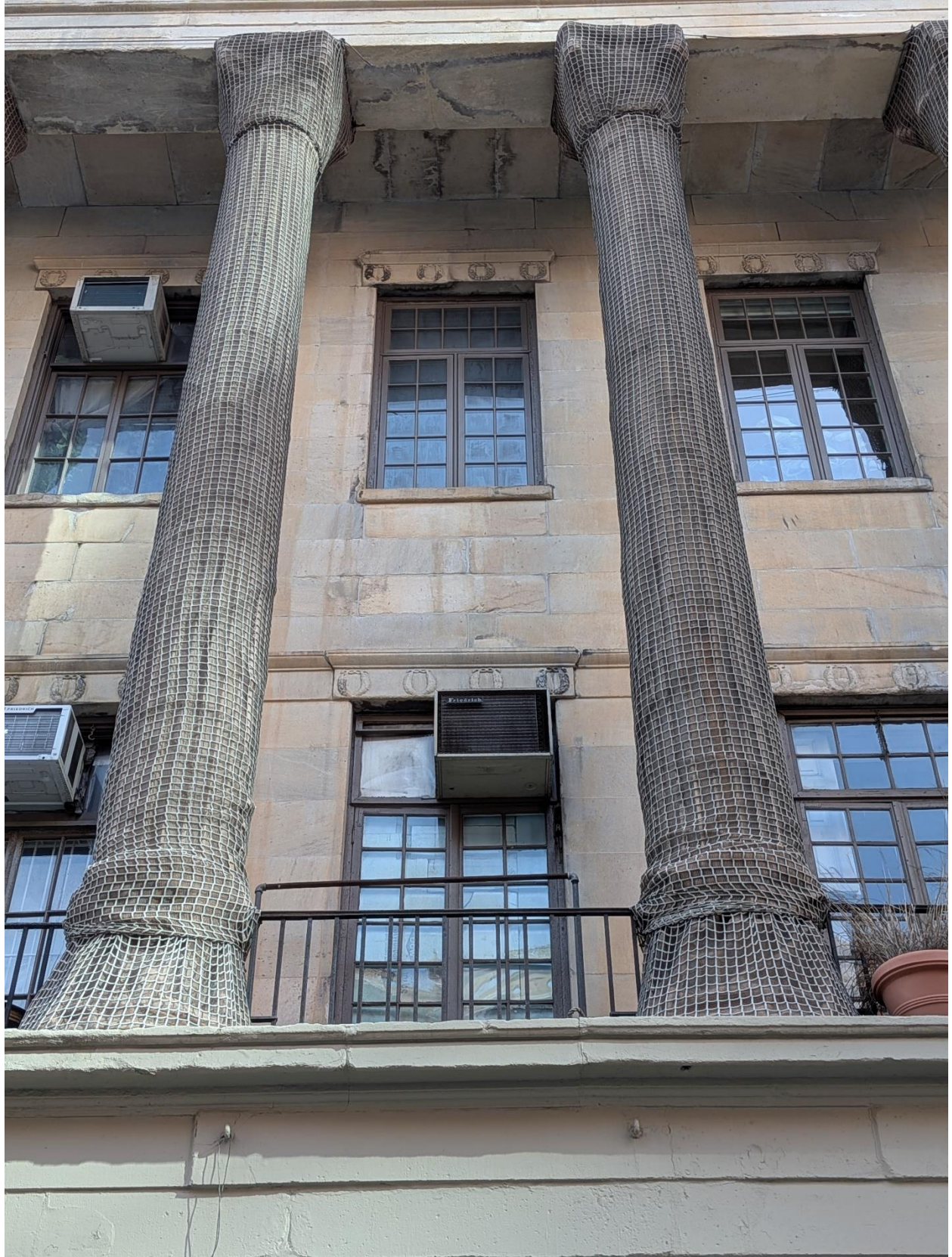
The marble façade is severely deteriorated. The columns have been wrapped in mesh for years.
