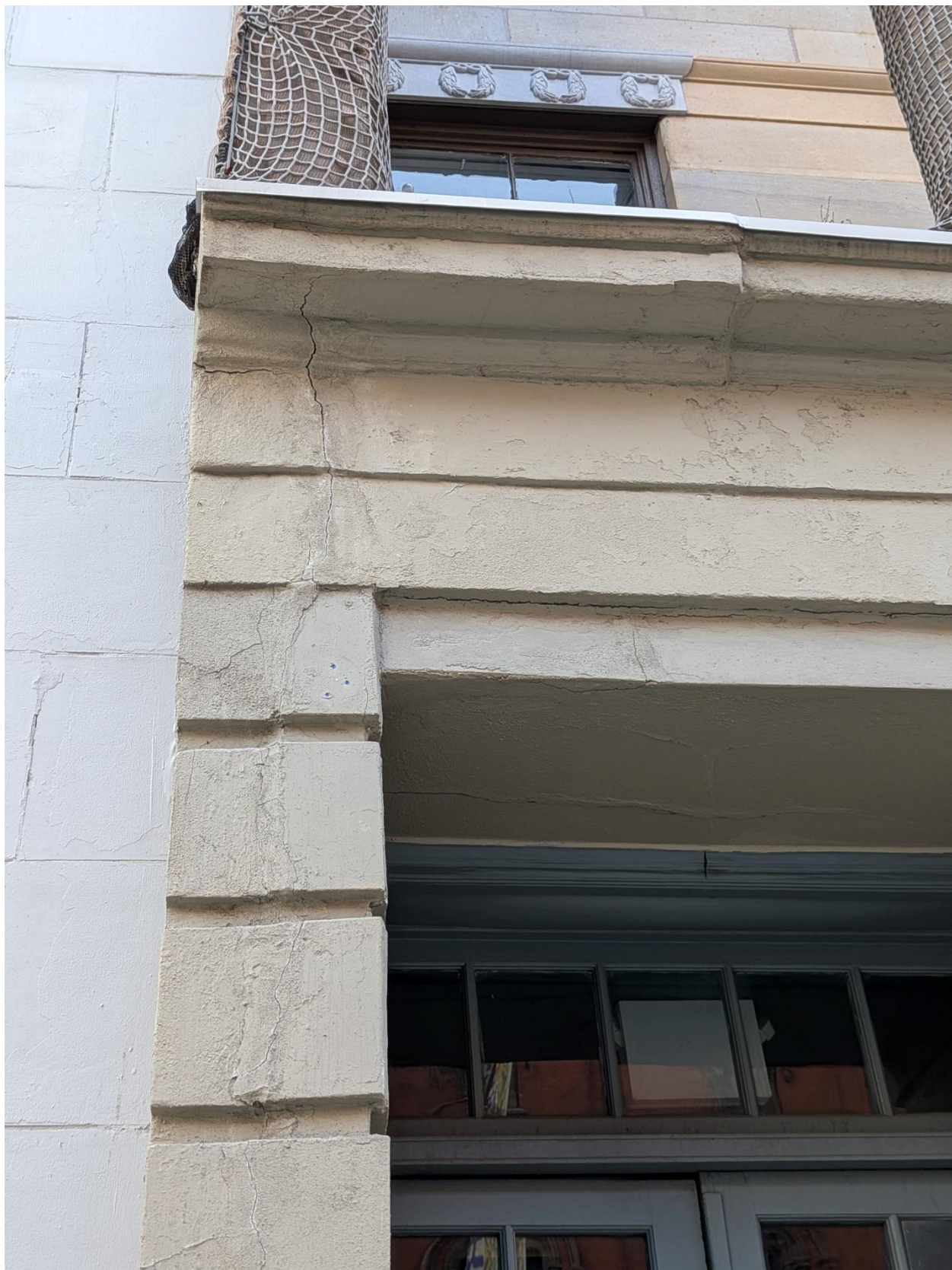
Additional conditions at the base of the buildings. The stone has been poorly patched and painted.
