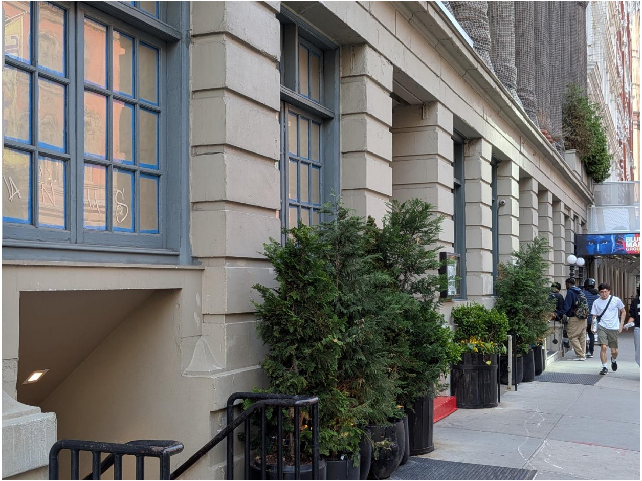
The relationship between masonry and window and door openings at the building's base is largely as it was originally.
