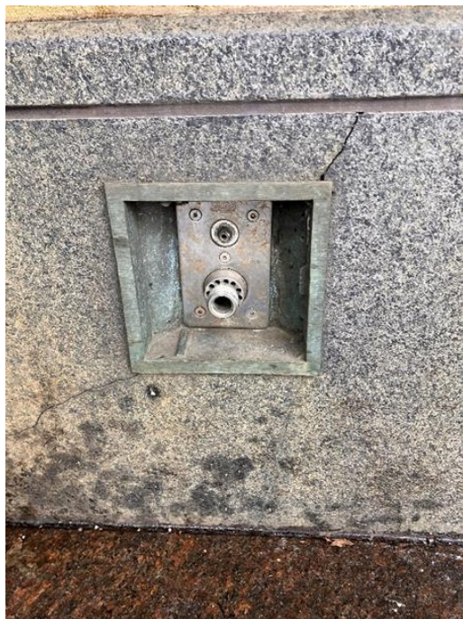
Hose bib on the south side of the station building. The missing cover shows the standard hose connection And valve. This hose bib is 40 feet from the scenic landmark.
