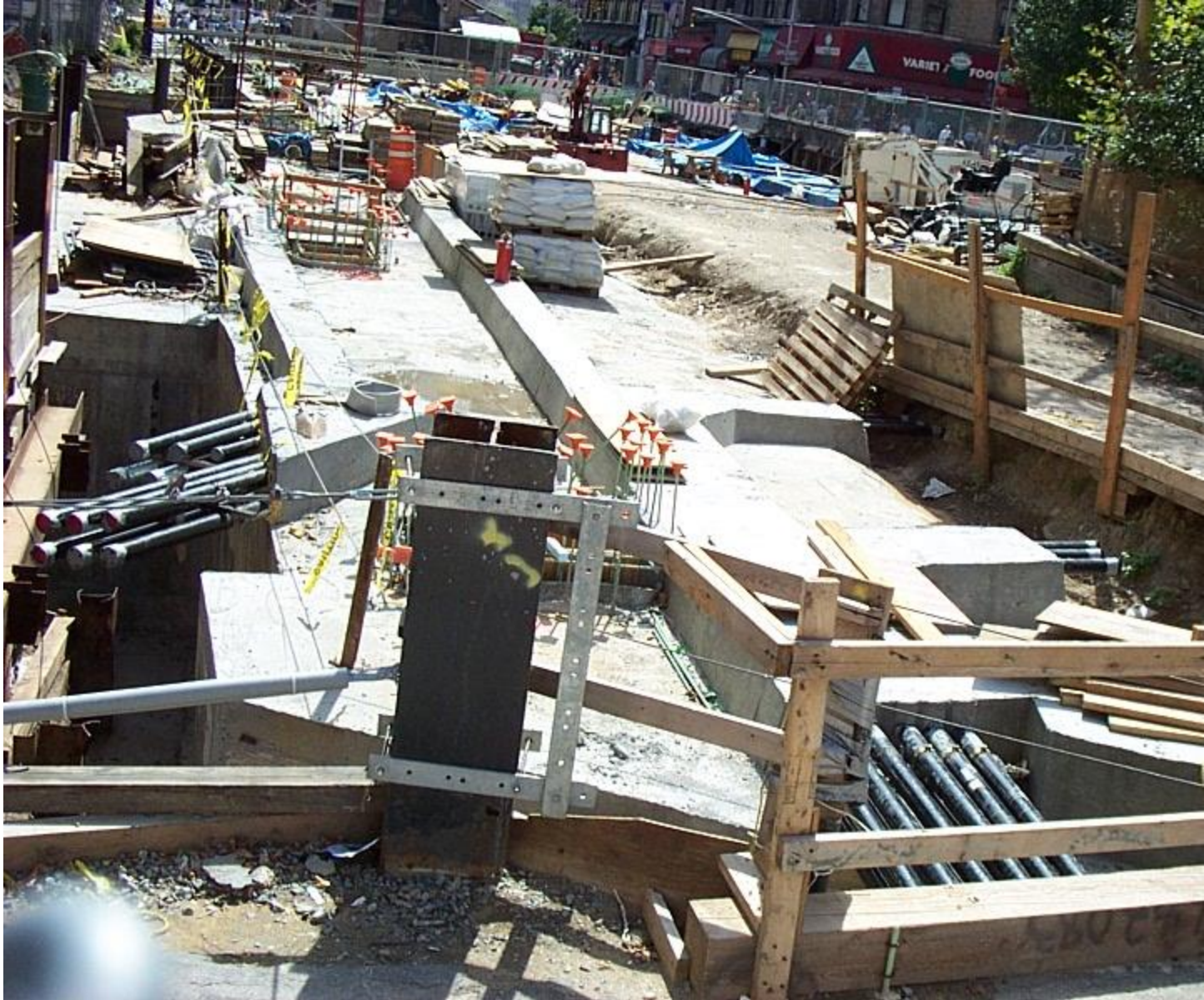
This image provides an idea of what is likely to be encountered if an attempt is made to install a new water line under the plaza pavement, which is directly above the subway tunnel and the old Broadway roadbed. This view by Michael Minn was taken during construction of the new control house, ca. early 2000's.
